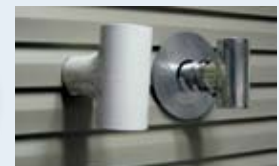
AL29-4C Stainless Steel Two-Pipe Venting
